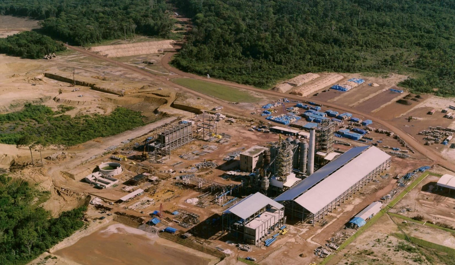
COSIPAR, Barcarena, Brazil, 2x 320 m 3 MINITEC Blast Furnaces.
